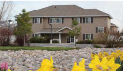
Built Outreach Office and Shelter -- 2002 & 2004
